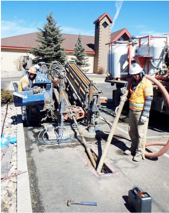
Pulling the fused 8" Pipe Under Valley View from Blackfoot Tr.
