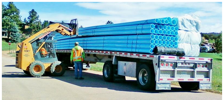
A delivery of 45foot long 4" 6" & 8" Fusible PVC Pipes
