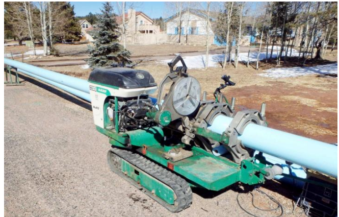
Fusing 8” pipe on Blackfoot Tr.
